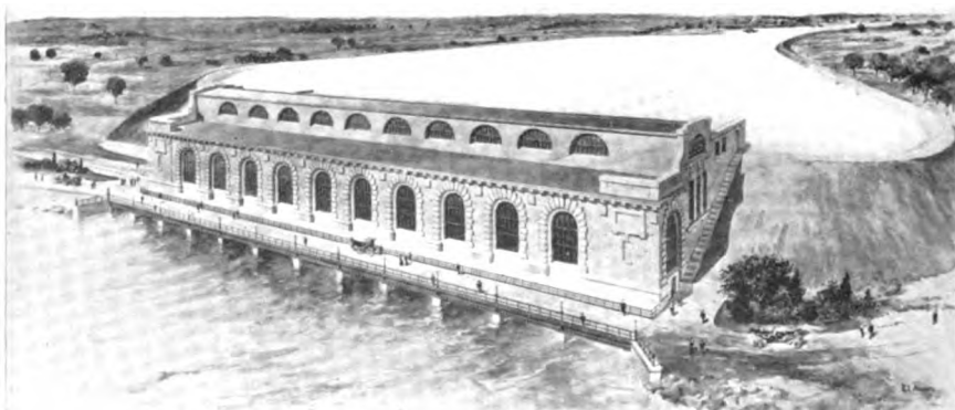
POWERHOUSE AND FOREBAY, THE CANADIAN LIGHT AND POWER COMPANY ST. TIMOTHEE, P. Q., NOW UNDER CONSTRUCTION
